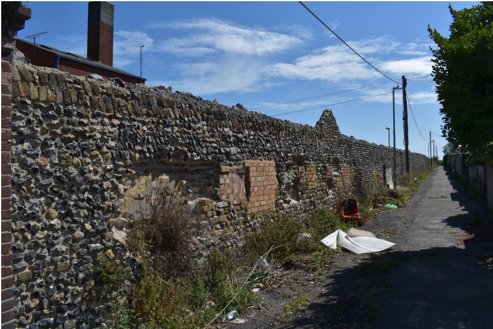
Plate 18: Southern side of the Bungaroosh wall from the public footpath (facing east)
